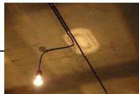
**03** Cable runs are fixed to the bare concrete ceiling with cable ties and self-adhesive pads of the kind used by electricians. Although this system is infinitely flexible, more permanent ceiling hardware may be installed in the future.
